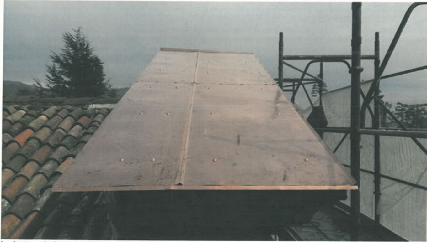
La lattoneria in rame a posa ultimata
